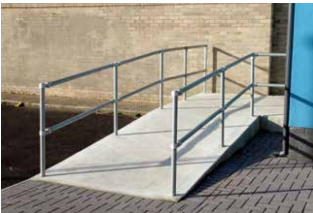
PIPE RAILING SYSTEM
